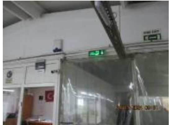
EMERGENCY_EXIT_WITH_BATTERY_LIGHT.JPG
